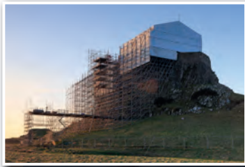
Layer scaffolding, Lindisfarne Castle, Scotland.
